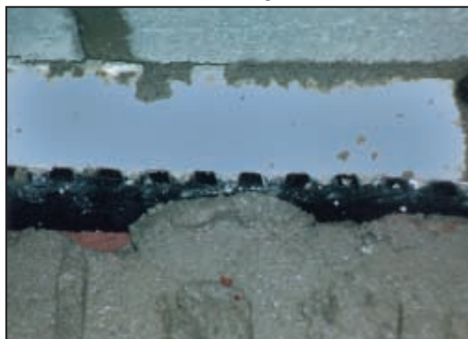
Figure 3 ThermaDrain ® stops mortar blockage.
