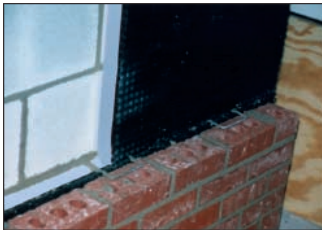
Figure 4 ThermaDrain ® is installed in easily handled board sections.
